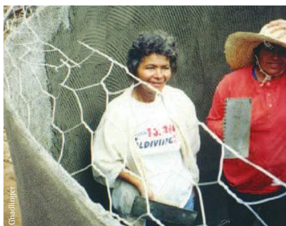
Lining a cistern with cement render
