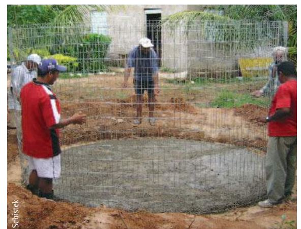
Constructing a cistern using self-supporting wire mesh
