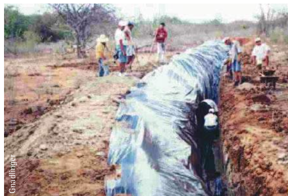
A PVC sheet is used to line a trench to minimise water loss
