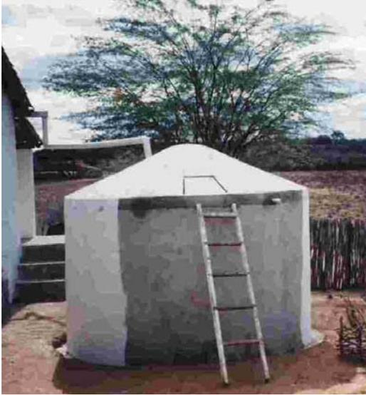
Illustration 3: 10 000 l wire-mesh concrete cistern
