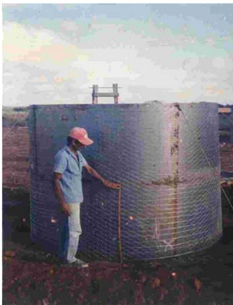
Illustration 5: Steel sheet form, wrapped by wire mesh and galvanized wire
