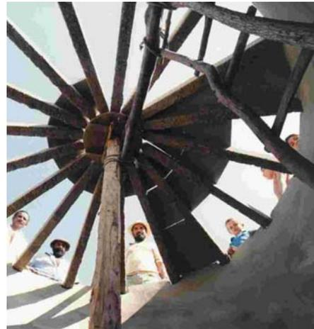
Illustration 2: *Process of covering the cistern (inside view)*
