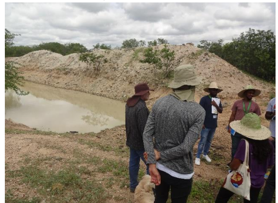
Four meters deep trench cistern of Mauri with water for sheep and goats
