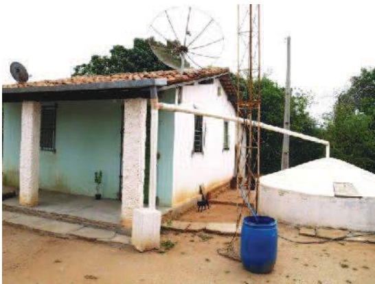
Figure 3 Plate tank at IRPAA Training Centre
